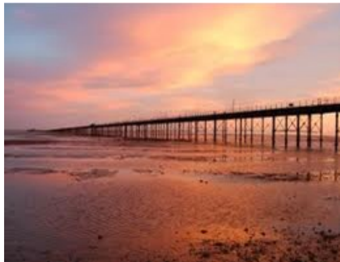
Southend Pier – still the longest in the world
